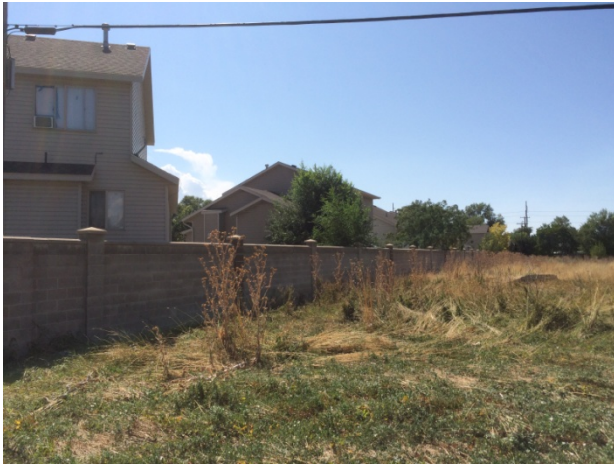
South wall and Justin Kay Court homes
